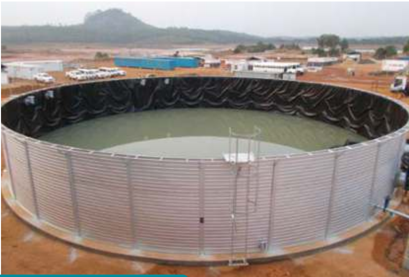
The completed ST30-03 (capacity of 1044 kℓ) during commissioning
