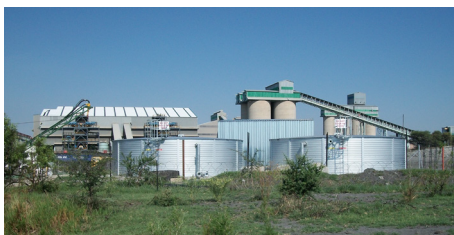
Mine infrastructure integration
